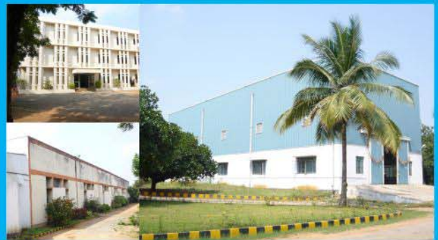
Hydraulic Cylinders & Naval Systems Plant
